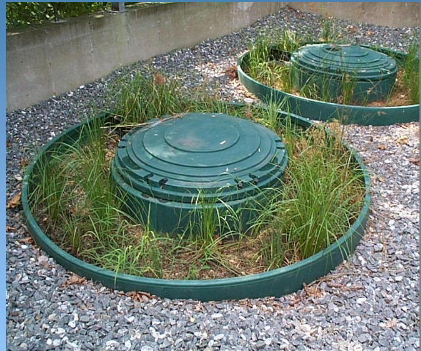
Cleaning Catch Basins
