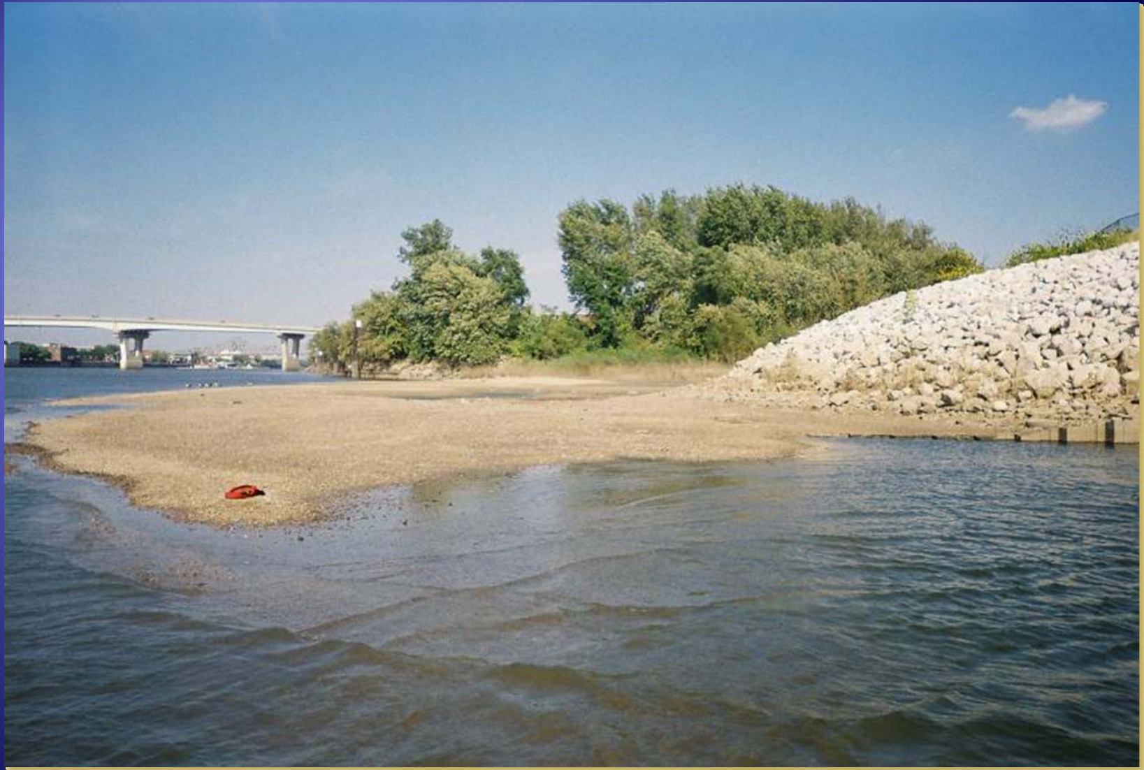
Farm Creek Channel Outlet to River
