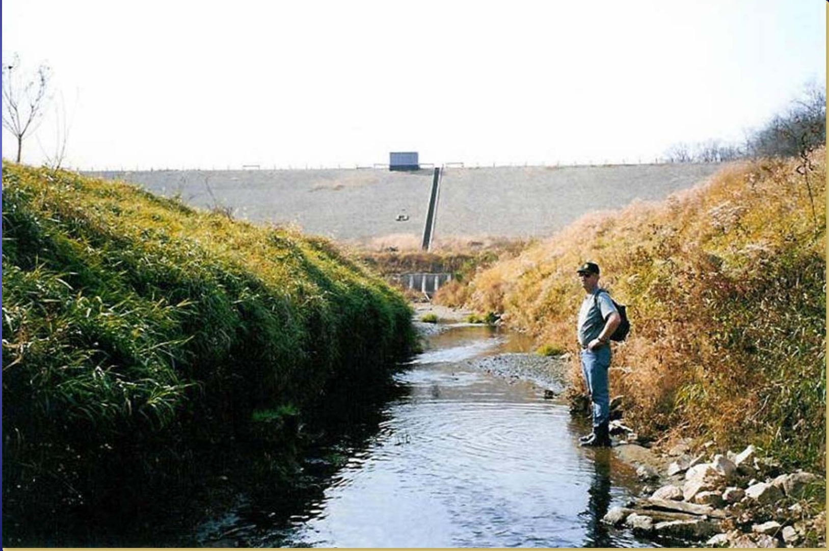
Enhanced Sediment Trapping in Flood Control Reservoirs
