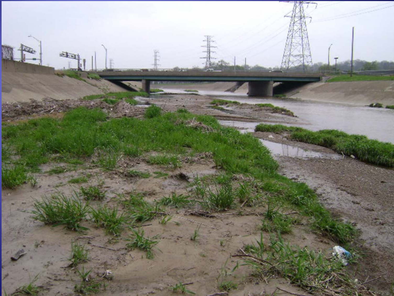
Farm Creek Channel at Main Street (IL 116) Bridge
