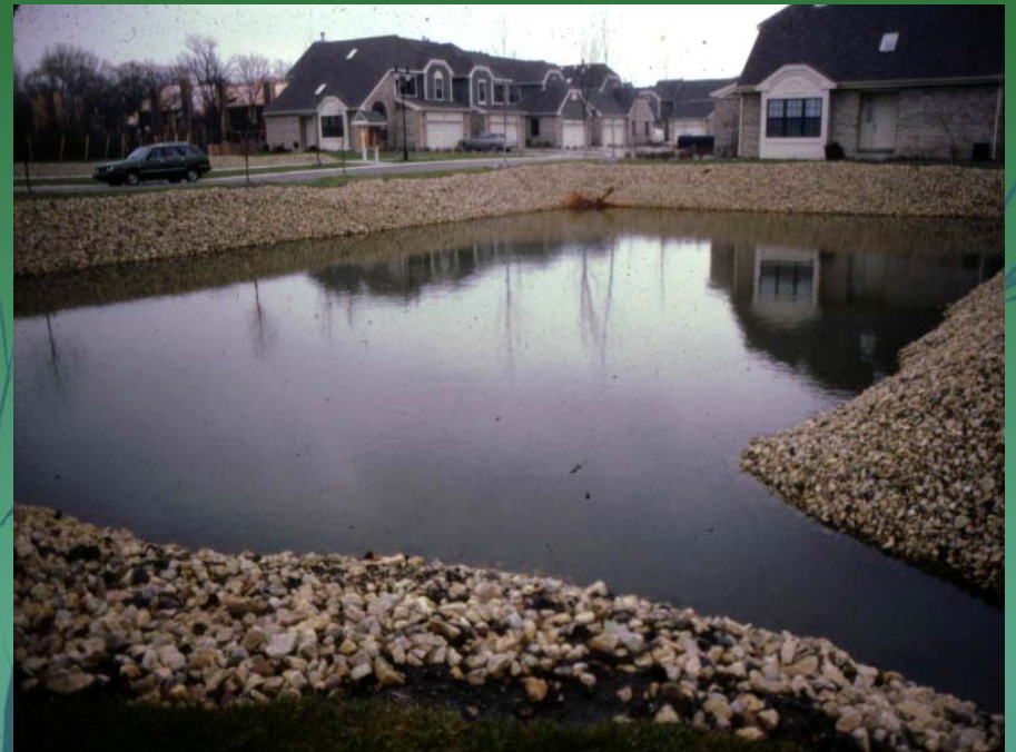
Traditional Detention Pond
