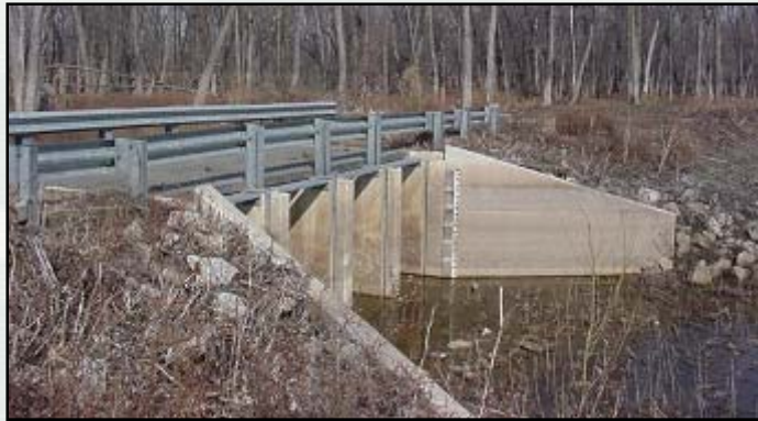
Water Control Structure
