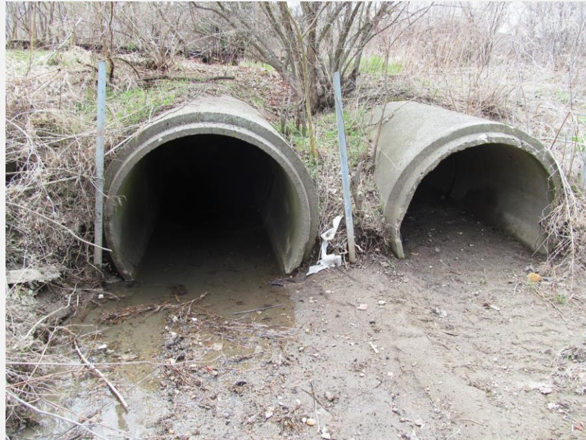
LACK OF MAINTENANCE CLEANING REDUCES CAPACITY
