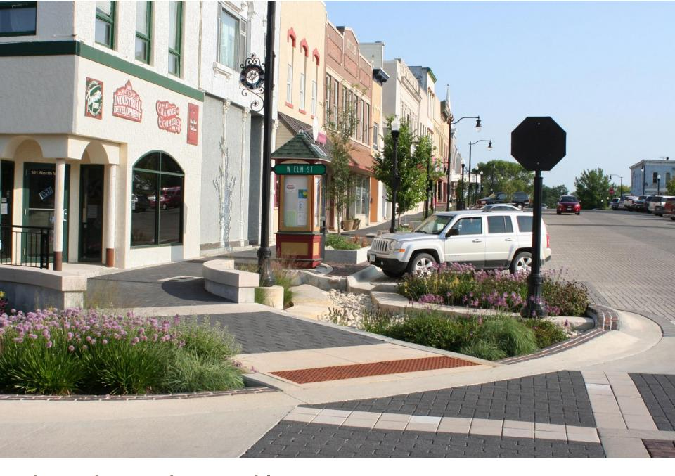
Rain gardens and permeable pavement to collect, infiltrate, and cool stormwater
